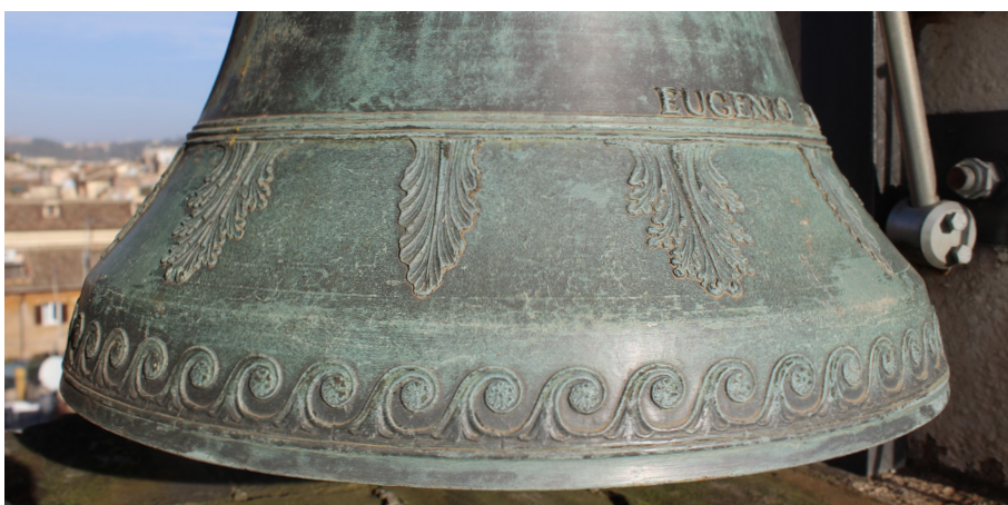
Fig. 26. Bottom part of bell no. 4. Both soundbow and rim are visible. The author
