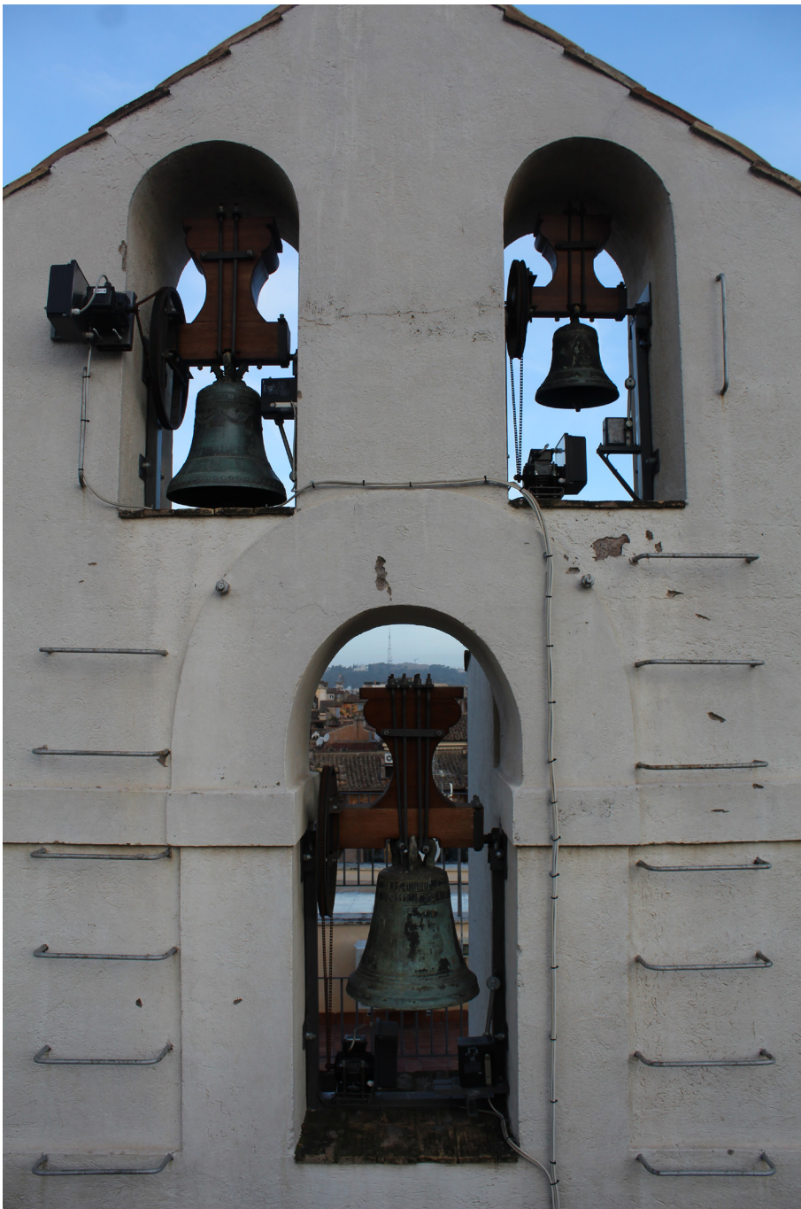
Fig. 4. The three bells on the top part of the bell gable. The author
