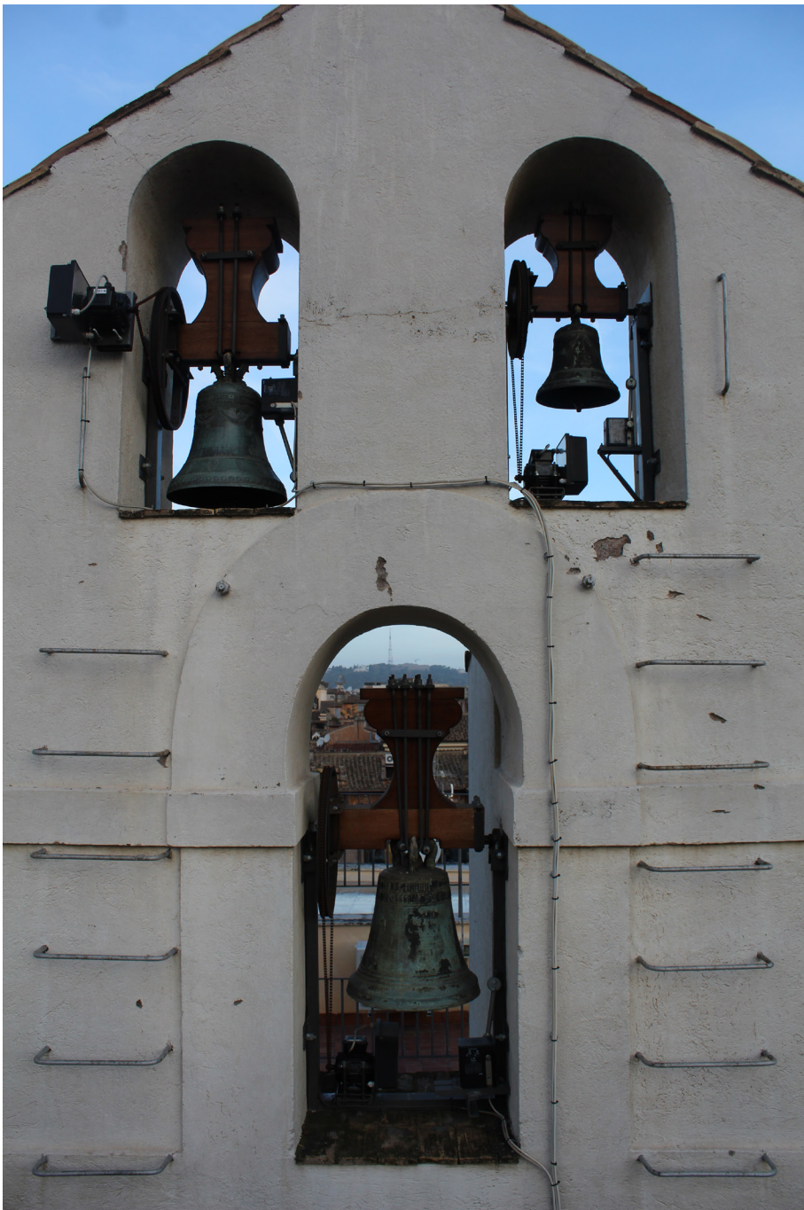
Fig. 4. The three bells on the top part of the bell gable. The author
