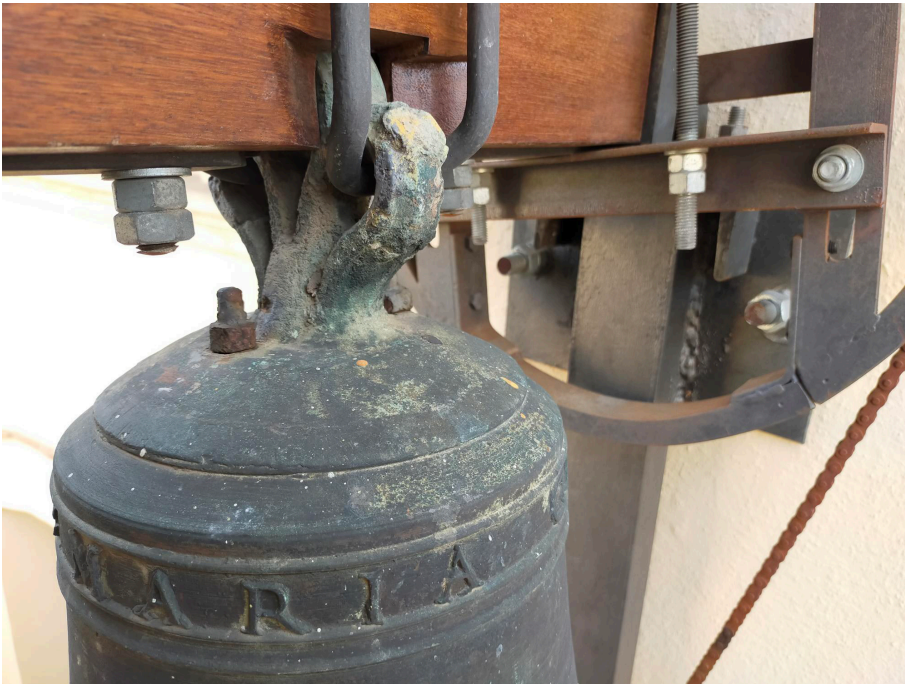
Fig. 11. Crown of bell no. 2. Part of the top inscription is also visible. The author
